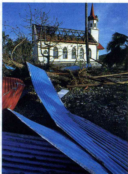
Damage from Cyclone Veena, Tahiti
