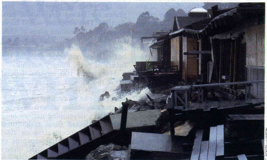
Beach residences collapse, Santa Cruz, California
